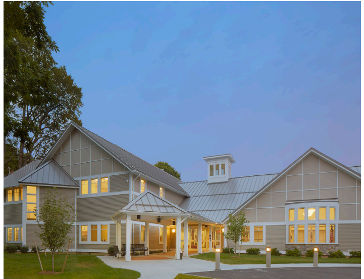
Marlborough Senior Center - Marlborough, MA
