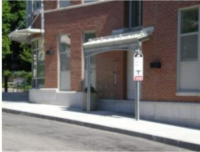
Figure 87 Integrated Bus Shelter in Belmont
