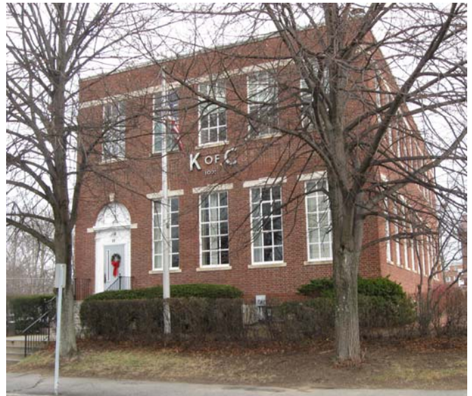
11 Sanborn Street, 1924. New England Telephone Switchboard Building
