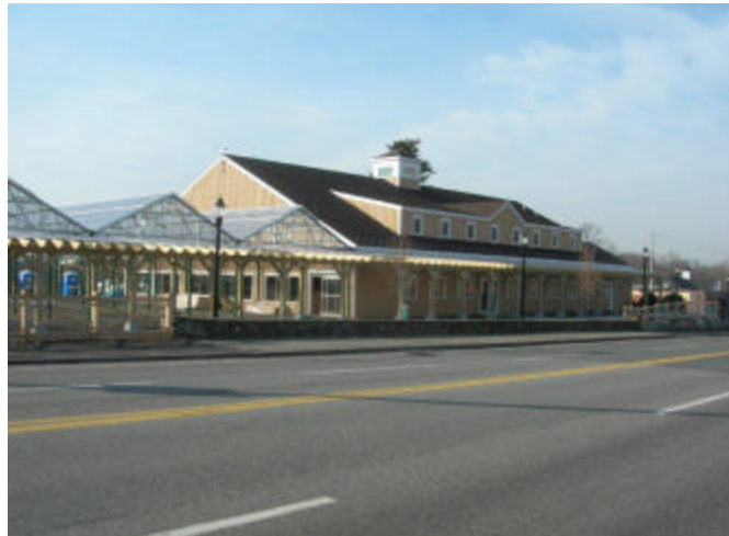
The NEW Calareso's is nearing completion!
