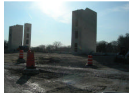
Construction of 1 st 50 Unit Bldg.
